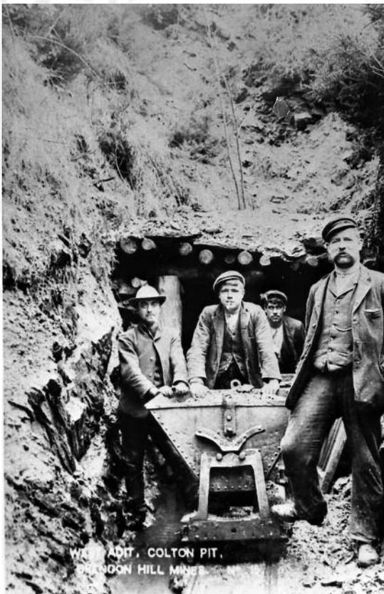
This photograph shows miners with a wagon of iron ore at the entrance to an adit when the mines were re-opened for the Somerset Mineral Syndicate in 1908. The miners are dressed rather smartly considering they are working underground. This is because they only would have had two pairs of clothes, one for every day, and one for Sunday best. The miner at the back of the picture is hunched over. The adit would have been dark, damp and cramped to work in. The photograph looks posed.
