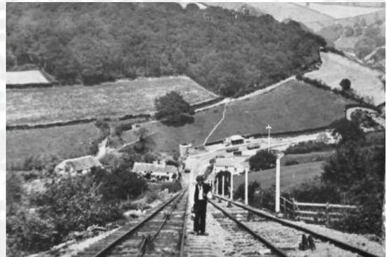
This photograph, taken in 1890, shows the view down the Incline from two thirds of the way down. The man has been identified as Jack Jewell, whose job it was every morning before breakfast to grease the railway rollers that carried the cables. He is carrying tallow on a stick to lubricate the rollers. The wooden poles carry wires for the semaphore signalling system between the top and the bottom.
