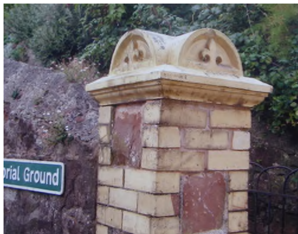
Pillar at the bottom of Goviers Lane, Watchet
